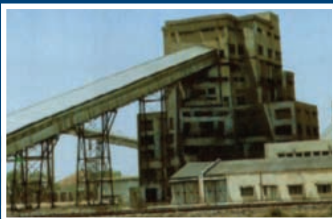
Coal Handling Plant, Paricha (UP)
